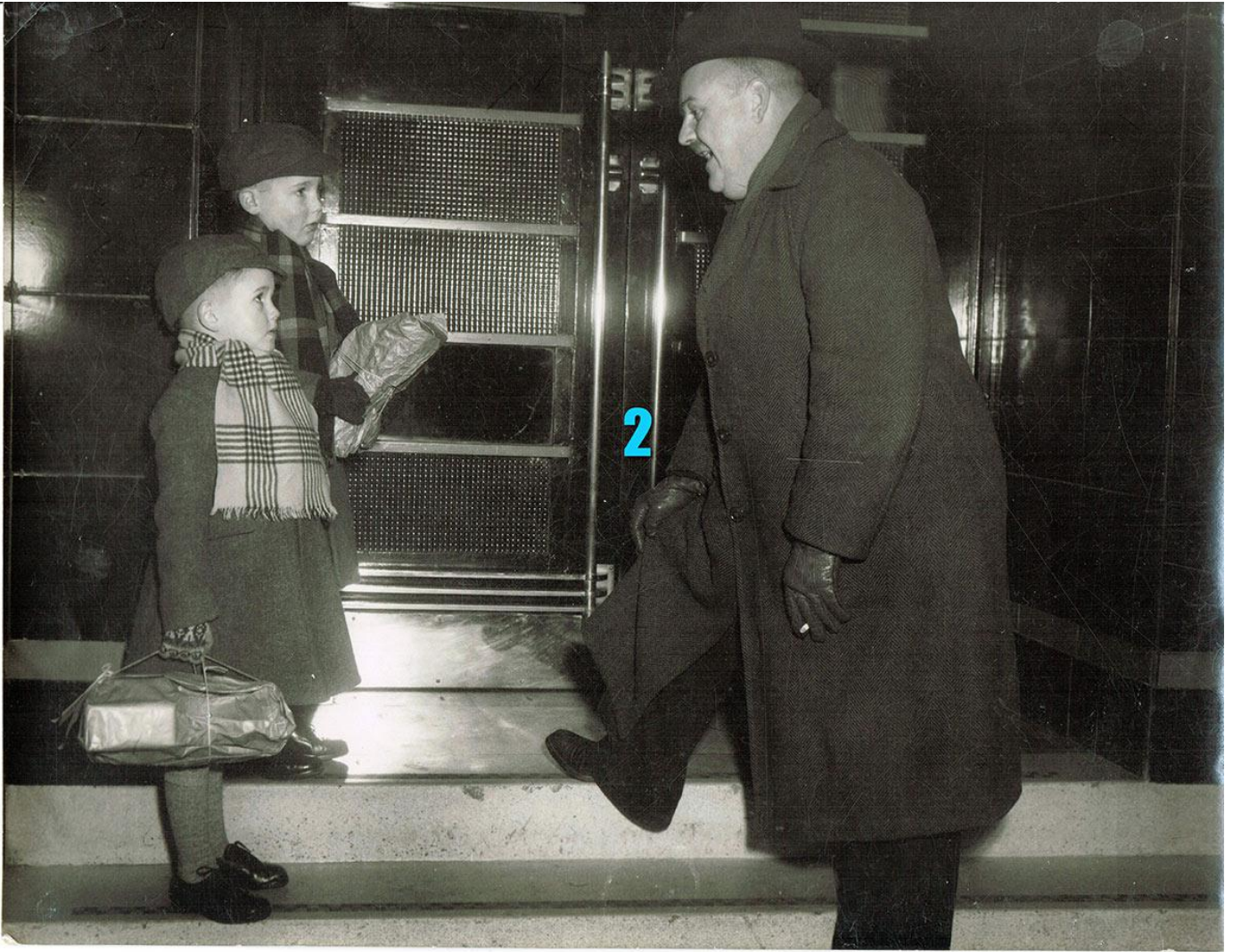
The original design Odeon fin doors with grand chrome handles, chrome kick-plates and 'Odeon glass'. We want to re-install all five pairs for a grand entrance. Two of these doorways are currently blocked by modern brickwork.
